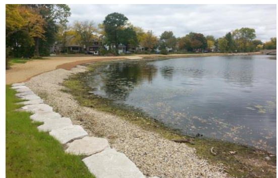
Photo of existing limestone wall at Tenney Park.
